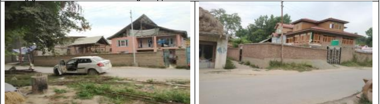
Left and Right Approach from the Dablepora side. Above 2 -3 houses stands at 90° with 35-40m distance from bridge approach road side. Proper installation of translucent view cutters (with standard height) at these points.
