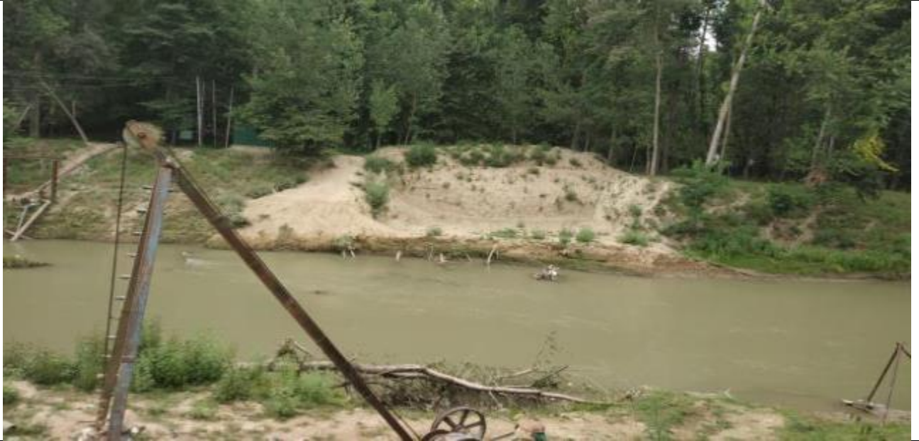
View of Proposed Bridge Site at Wachi from RHS side (Dablepora)
